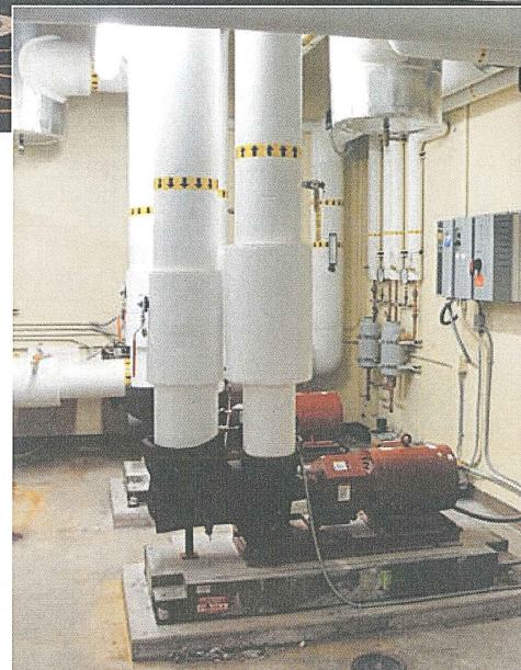
ABOVE: Bell & Gossett model 1510 base-mounted pumps and Tech 502 variable-speed system to optimize pumping efficiency.
